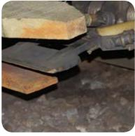
At some places there is a pick-up rail which is not protected. This is marked as shown above. At such points it is not allowed to step over the third rail.
