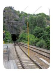
The third rail contains 700 V DC and the catenary 1500 V DC. If a catenary has fallen down or got broken in some way do not touch it.
